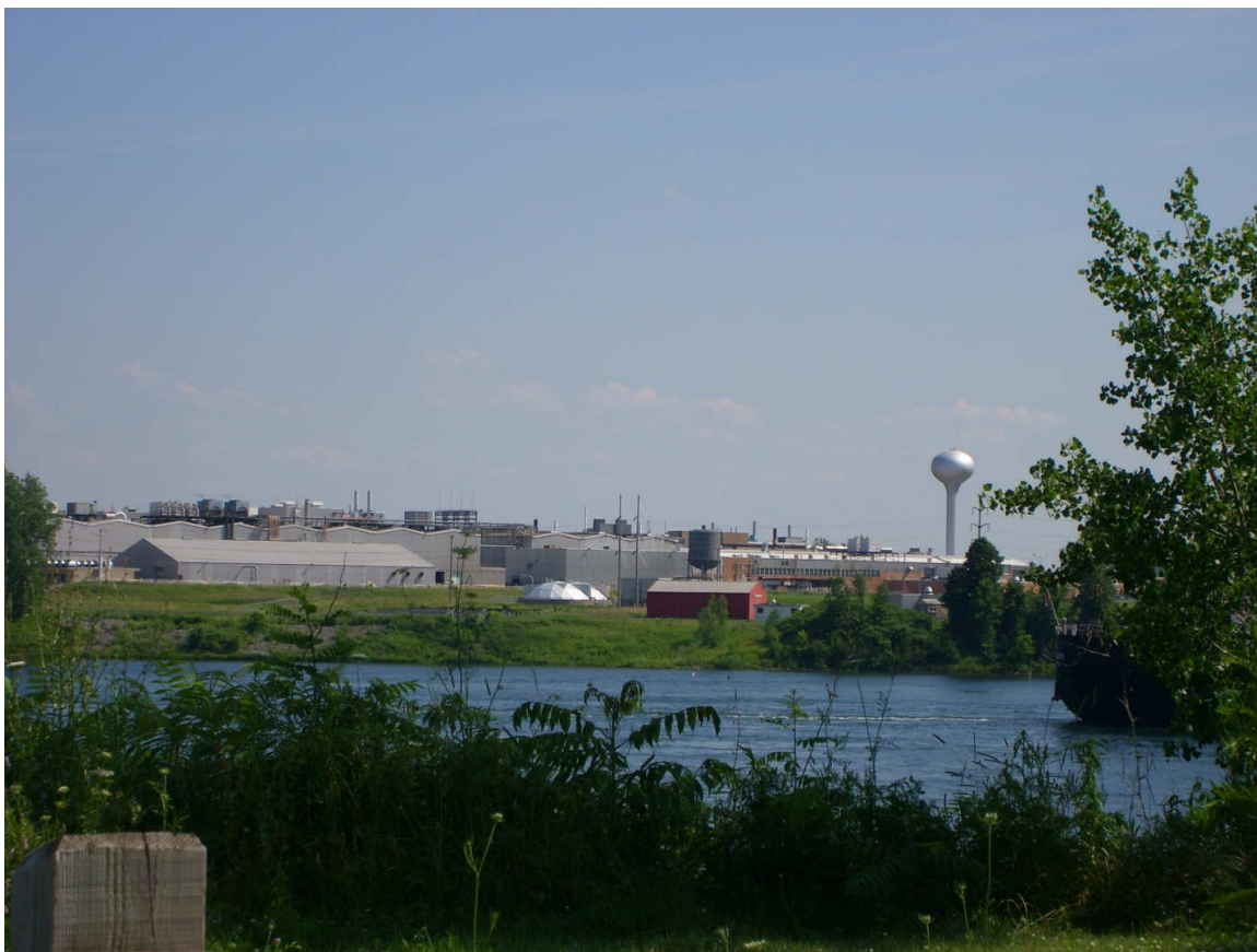
View of General Motors Central Foundry from Gina's front yard
