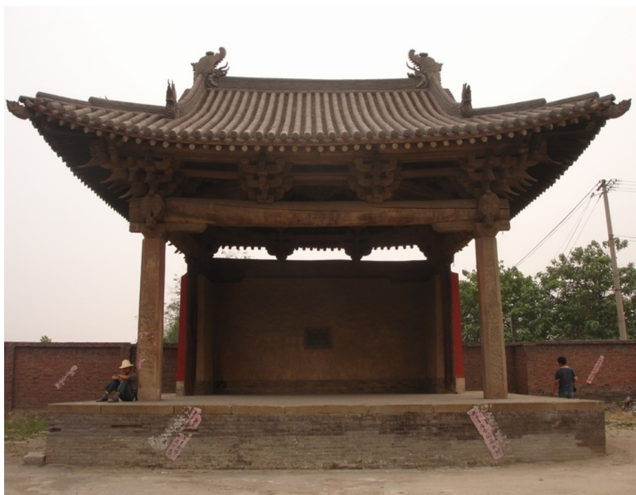
Figure 4.21 The Yuan-dynasty stage at the Niuwang Temple, Weicun village, Linfen county, construction during 1283-1321 (Photo by , 08/2009 Zhang).
