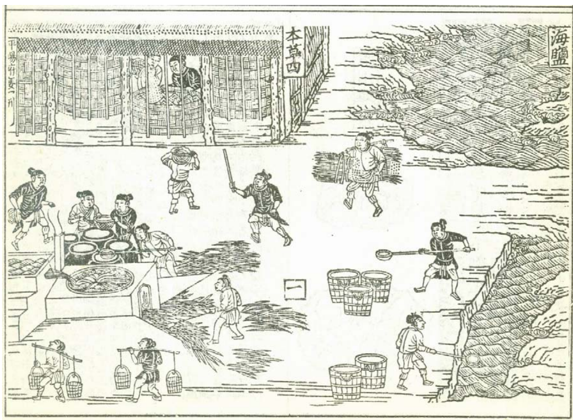
Figure 1.12 Illustration of the process of making sea salt, the Materia Medica , 1249, juan 4, 104b.
