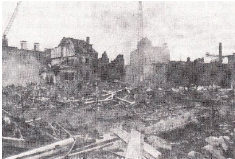
Figs. 1.6-1.7, Photographs showing the West End before and after demolition In: O'Connor, Building a New Boston , 1995
