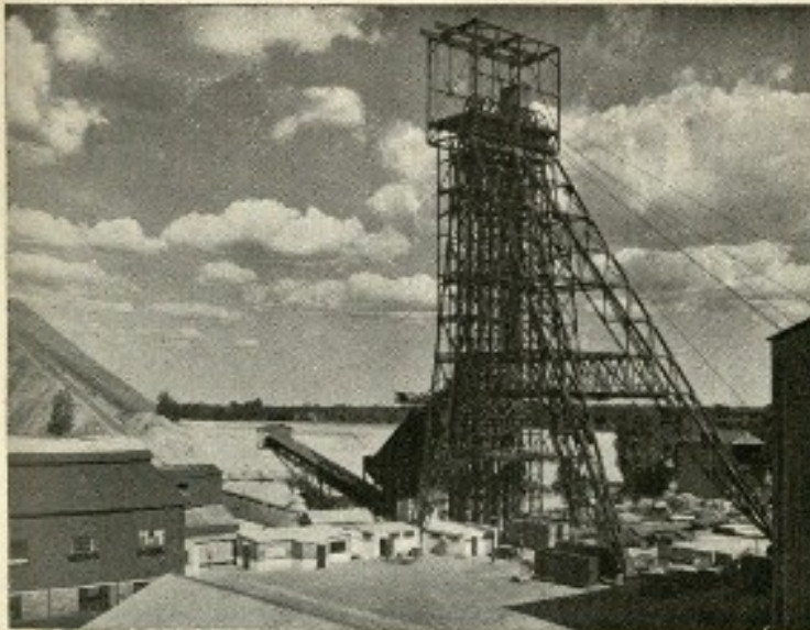
Typical headgear of a gold mine
