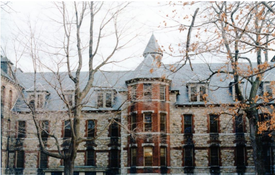
Figure 34. The second Worcester State Hospital showing the decorative effects of the contrast between the “rough ashlar stone” used in the main body of the building and its brick trimmings. Photograph by Paul Rohde, 1983. Worcester Historical Museum, Worcester, Mass.
