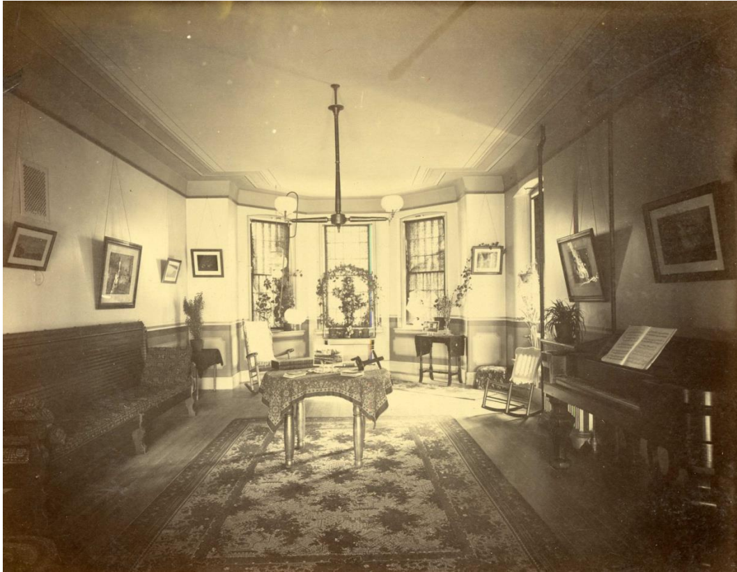
Figure 17. Ward in the second Worcester State Hospital (undated; late 19 th century), showing many of the features Woodward described in the “better” wards of the first hospital, including a piano, pictures, spaces for recreational activities, and abundant light. A stereoscope and pictures are available on the center table for patients’ amusement. Worcester Historical Museum, Worcester, Mass.
