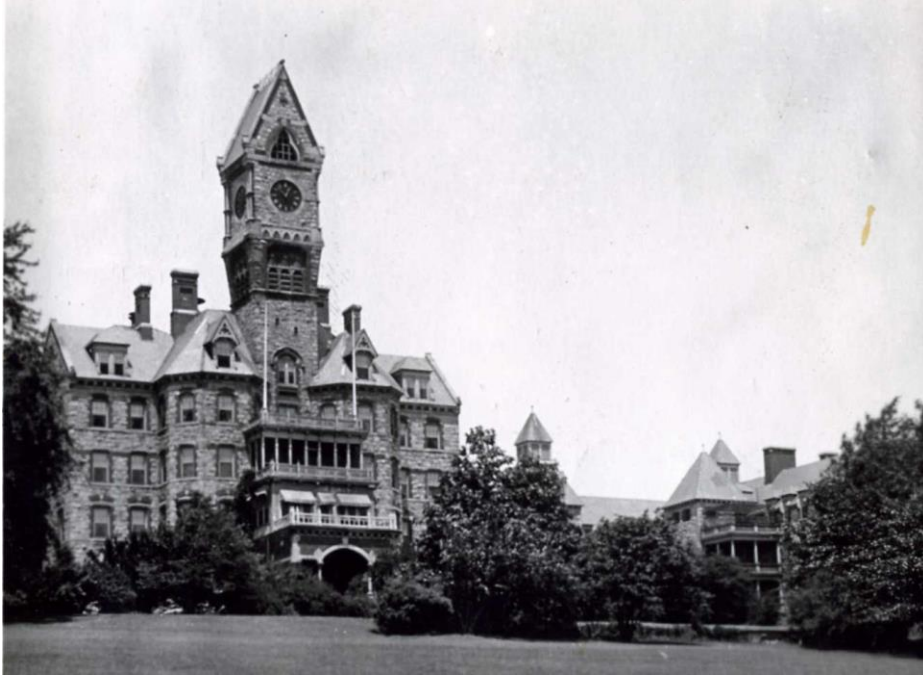
Figure 33. The Gothic façade of the second Worcester State Hospital (undated; late 19 th or early 20 th century). The cupolas were decorative elements used to disguise ventilation shafts. Worcester Historical Museum, Worcester, Mass.
