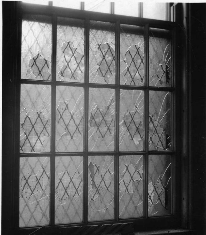
Figure 18. Window at the second Worcester State Hospital showing panes broken by a patient. Undated photograph, Worcester Historical Museum, Worcester, Mass.
