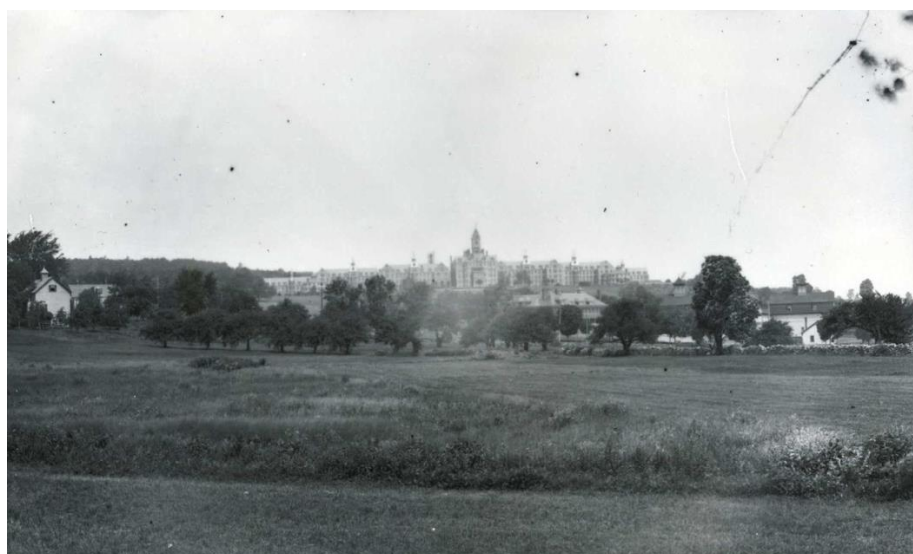
Figure 13. The second Worcester State Hospital, circa 1900. The main complex (with central clock tower and branching wings) is in the background of the photo, at the top of the hill. The buildings in the foreground belong to the asylum farm. Worcester Historical Museum, Worcester, Mass.
