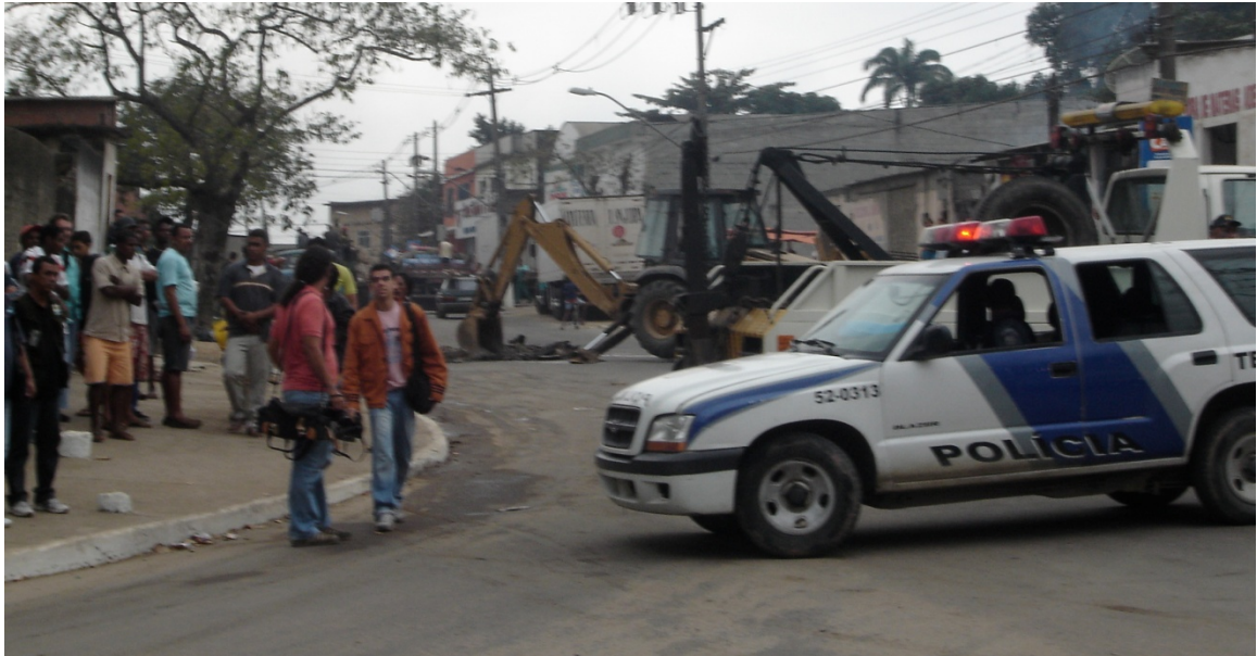
Figure 2.8 A bulldozer breaks up the road on Avenida Monte Castelo as police arrive and a crowd gathers.
