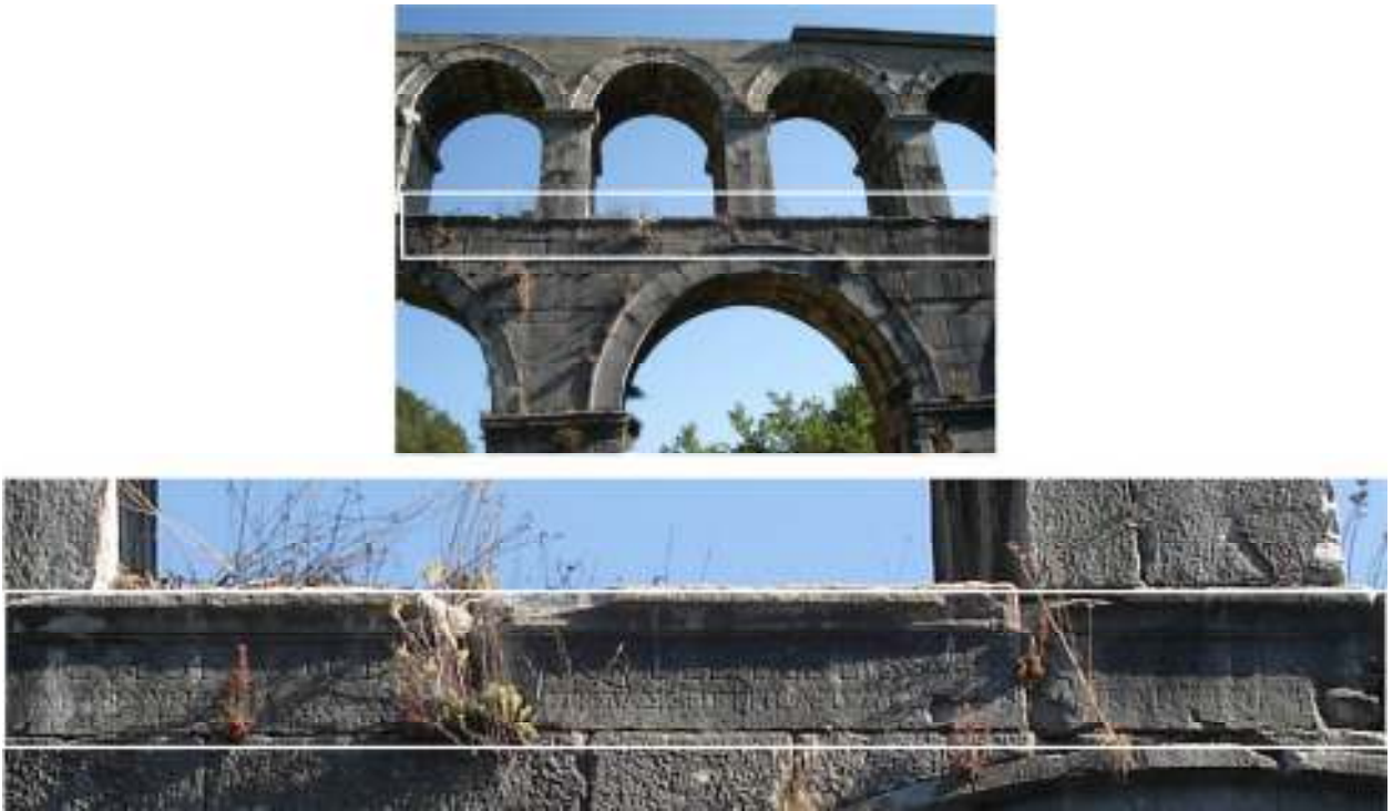
Fig. 3.11 Pollio Aqueduct Bridge (above) and detail of dedicatory inscription (below) (author photo)
