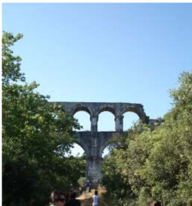
Fig. 3.10 Pollio Aqueduct Bridge, Ephesos (Augustan, 27 BCE – 14 CE) (author photo)
