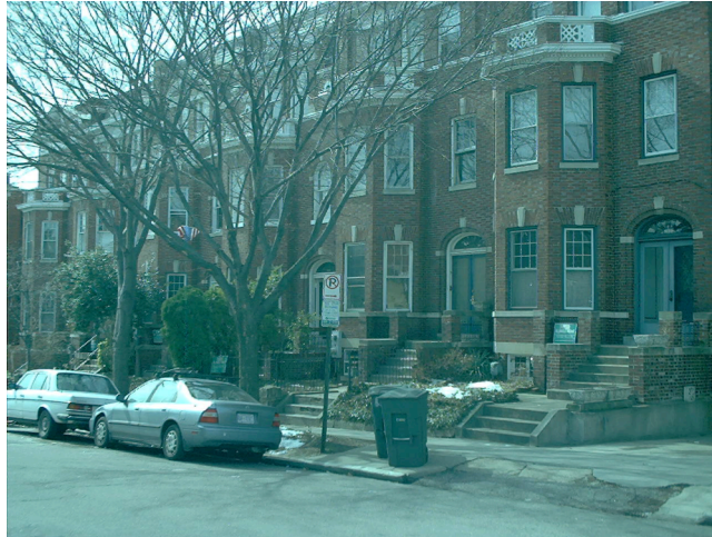
Figure 3: A row of houses, 17th Street, Mount Pleasant, February 2005
