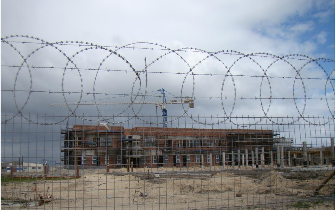
Khayelitsha Hospital under construction (Source: Amy Kracker Selzer 2010).
