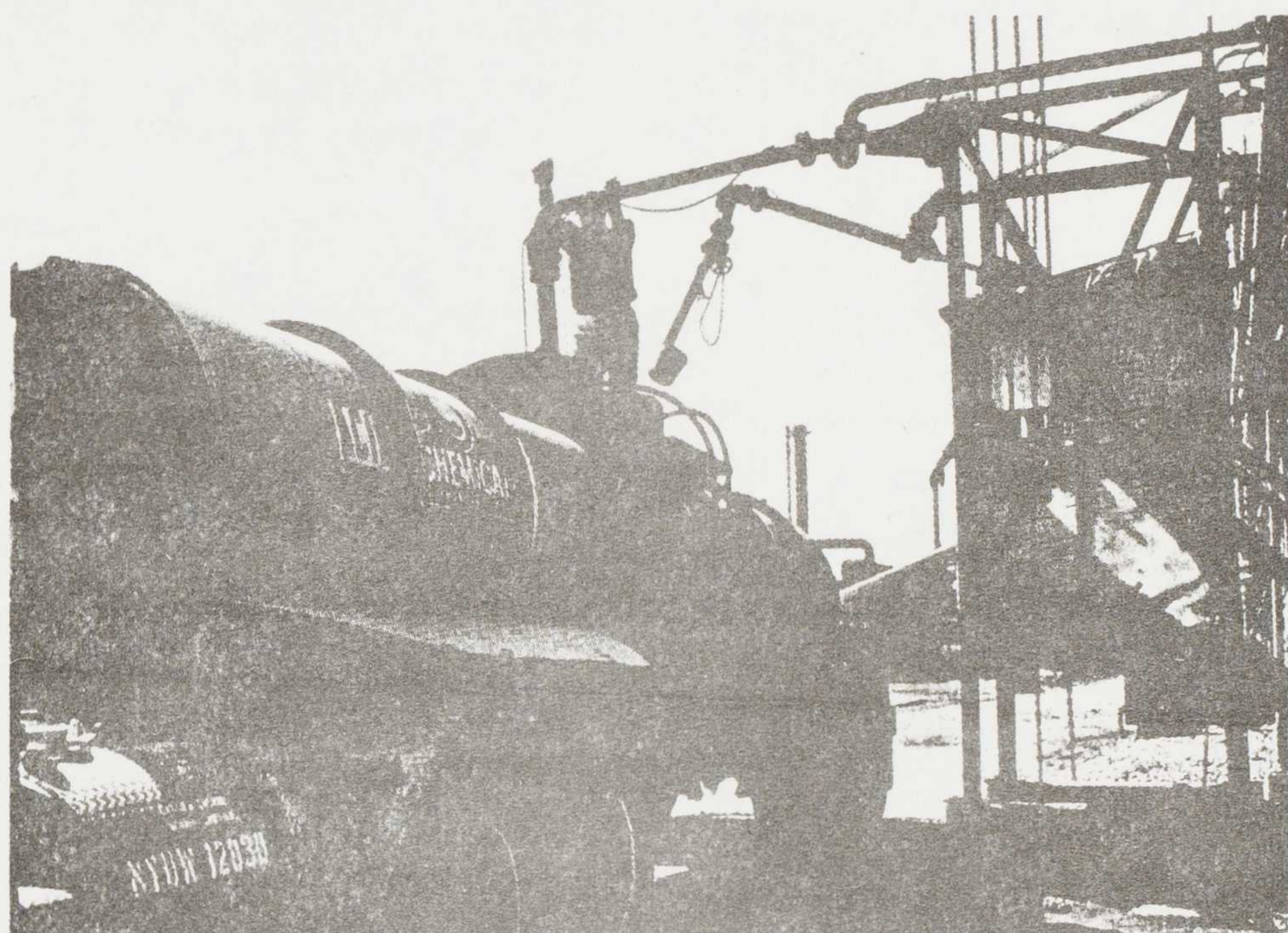
Road tankers deliver hydrofluosilicic acid to cities which use it to fluoridate water. Tanker is typical of the many that are rubber-lined by our Chemical Plant Division.
