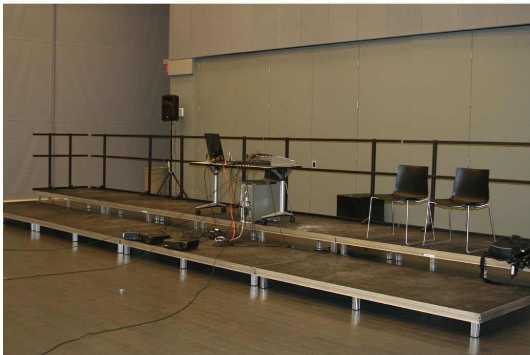
Figure 12. The tiered seating and mixing position being installed.
