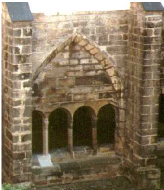
Fig. 105. Cloister, east aisle exterior arcade.
