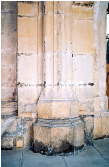
Fig. 107. Cloister, east aisle, interior wall responds.
