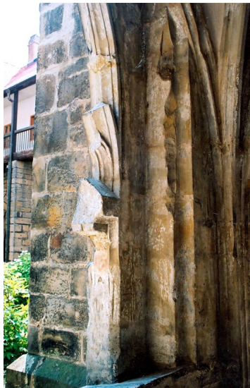
Fig. 123. Cloister north aisle.
