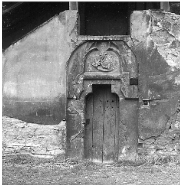
Fig. 17. Litovice, near Prague, portal.
