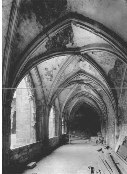
Fig. 102. Cloister, west aisle, interior, view south.
