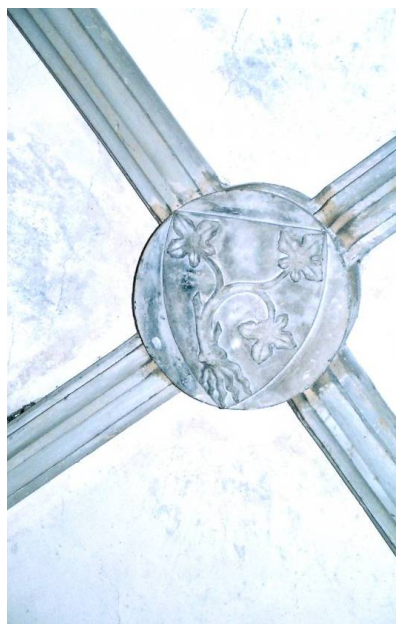
Fig. 84. Vaulting boss, Chapter room.
