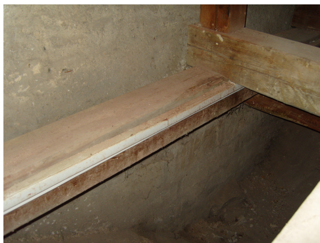
Fig. 93. Roudnice monastery, above south church aisle, nave wall.
