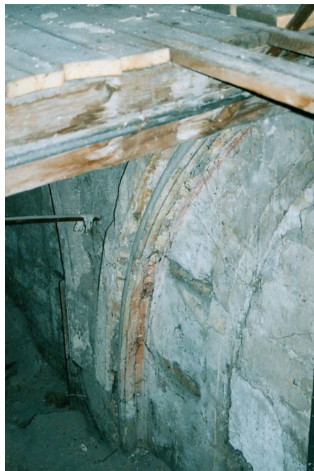
Fig. 92. Roudnice monastery, above south church aisle, nave wall.
