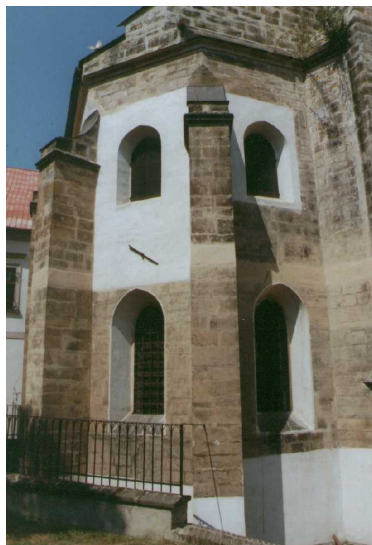
Fig. 61. Roudnice monastery, sacristy and upper storey, exterior.
