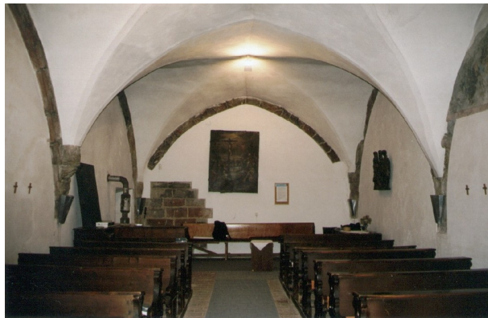
Fig. 73. Upper story of sacristy, west end.
