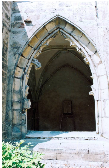
Fig. 122. Cloister north aisle.
