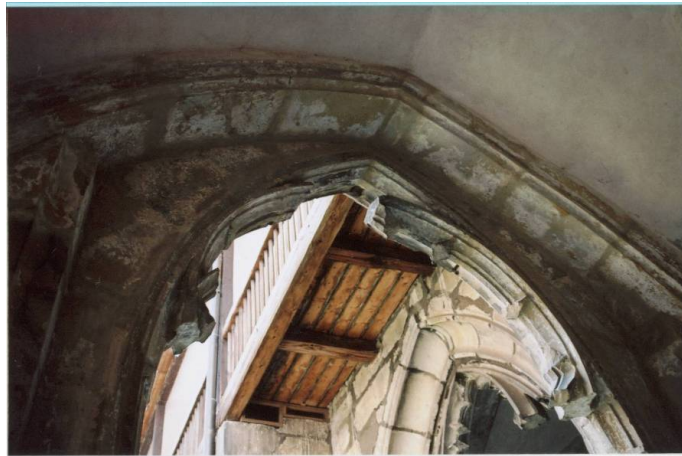
Fig. 121. Cloister north aisle.
