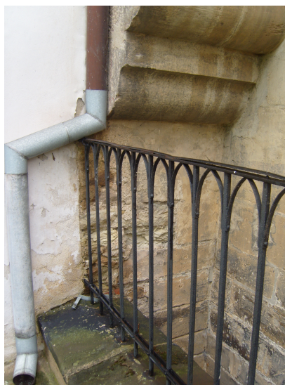
Fig. 62. Roudnice monastery, border of sacristy and chapter room, exterior.
