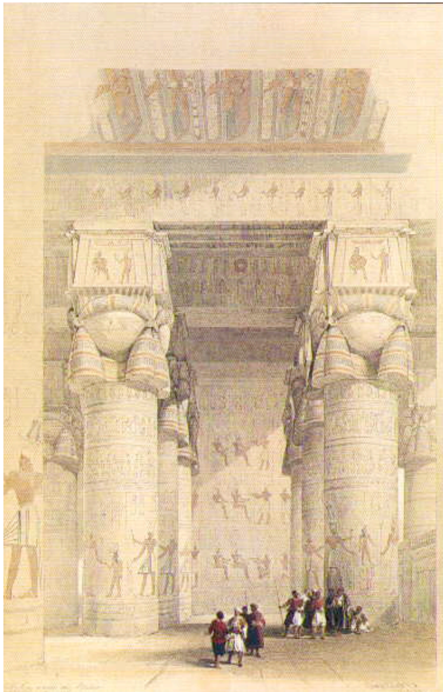
6. View under the Portico, Dendera (1842)
