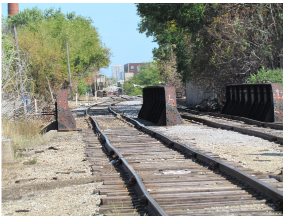
Figure 3.10: Bloomingdale Trail, looking toward the terminus, Fall 2011
