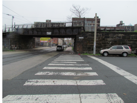
Figure 3.13: Reading Viaduct from street level, Spring 2011
