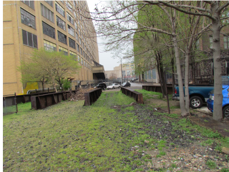
Figure 3.12: Reading Viaduct entrance at grade, looking toward Spring Garden, Spring 2011
