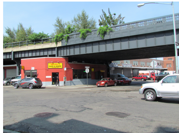
Figure 3.5: View of High Line from across 10 th Avenue, Summer 2011
