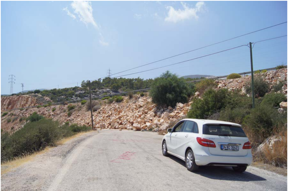
Fig. 5.3. West of Taşucu (ancient Holmoi). The old coast road has been blocked by the construction of the new highway (above).
