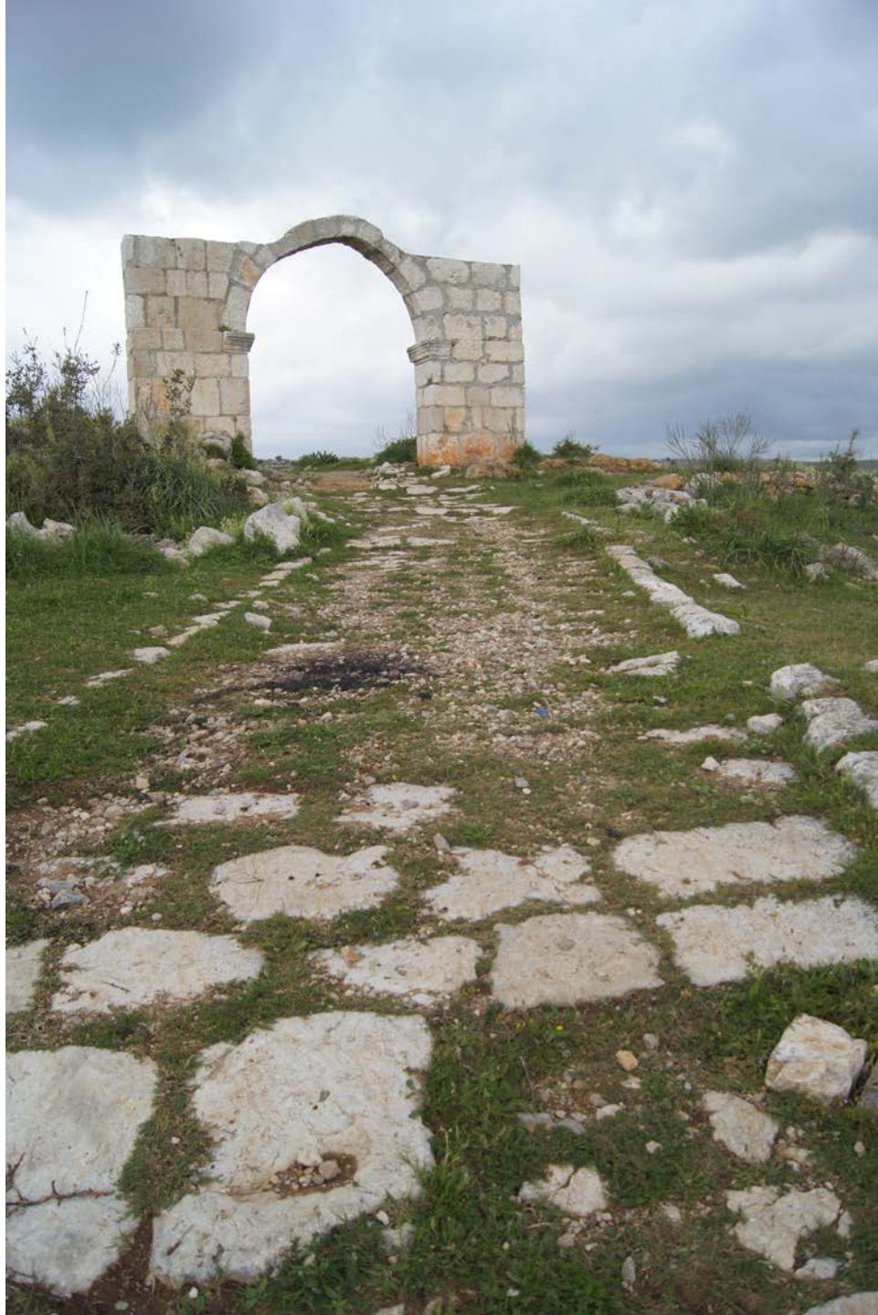
Fig. 5.5. The paved Roman road north of Tarsos on the via Tauri, at the monumental arch (near modern Sağlıklı), with visible paving stones and kerbs.
