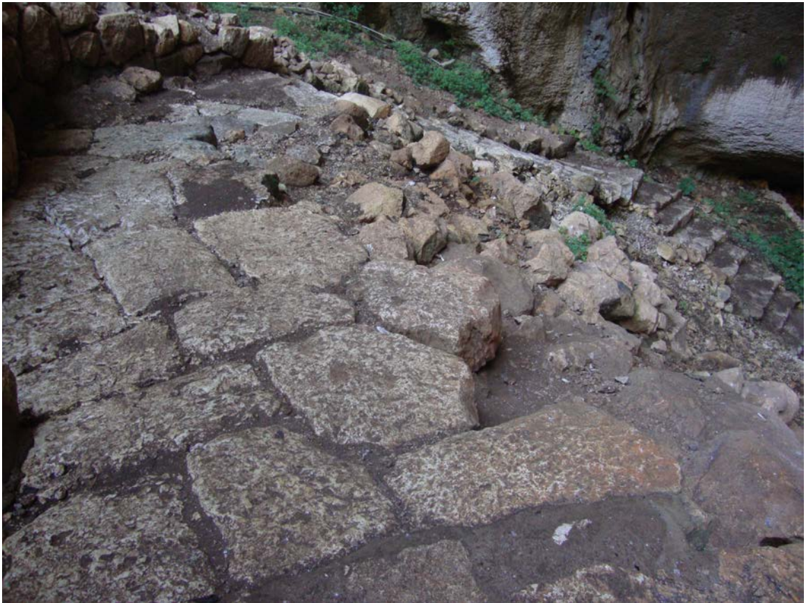
Fig. 4.15. Korykion Antron (modern Cennet Cehennem). Staircase descending from the Chapel of St Mary, at the far southern end of the depression 'Heaven' (Cennet) into the cave.
