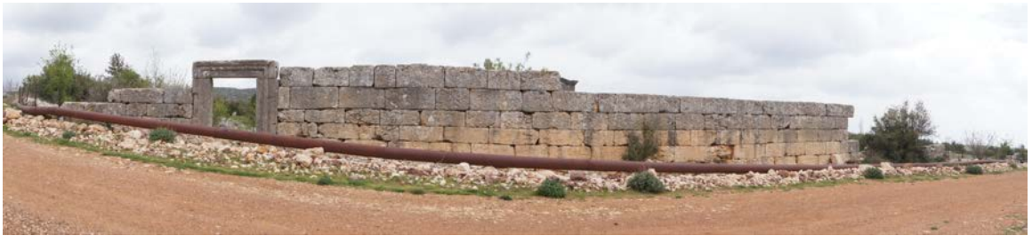
Fig. 5.19. Cambazlı. The western (main) gate in the church precinct.
