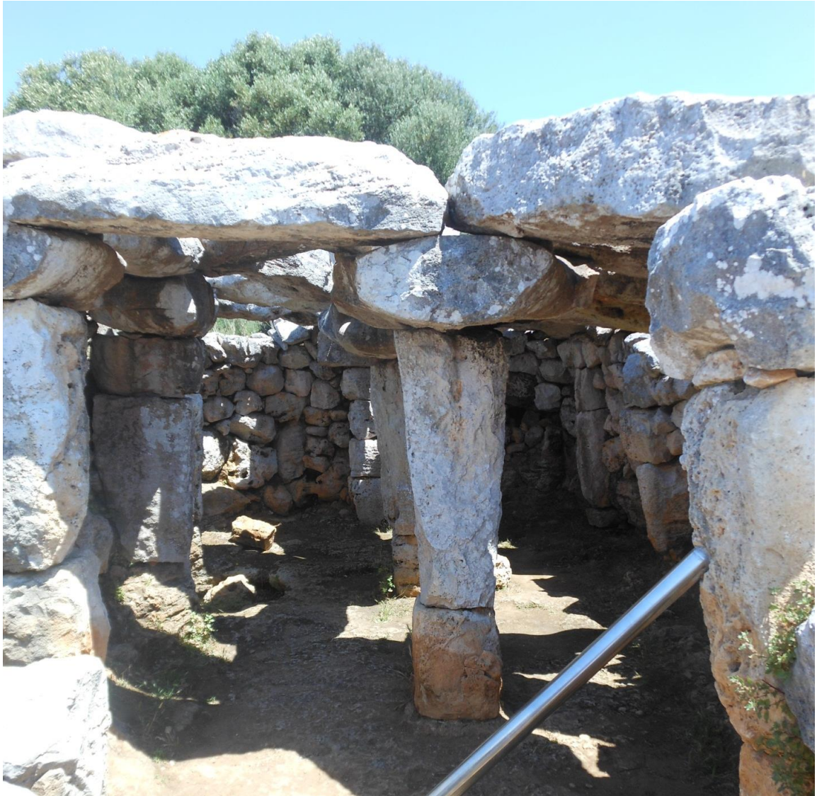
Figure 45: Hypostyle hall of House 6 at Torre d'en Galmés in 2014. The hall is actually roofed with megalithic limestone blocks, and was most likely used as a storage facility. (Photo by the author)
