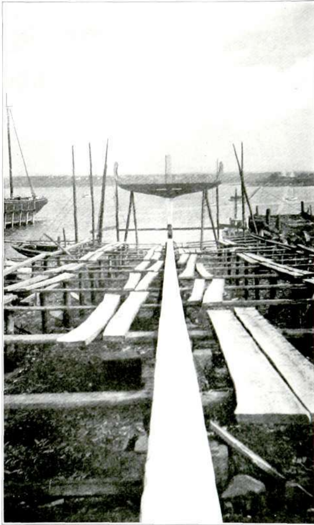
A newly laid keel at the Snow yard, Rockland, Maine.
