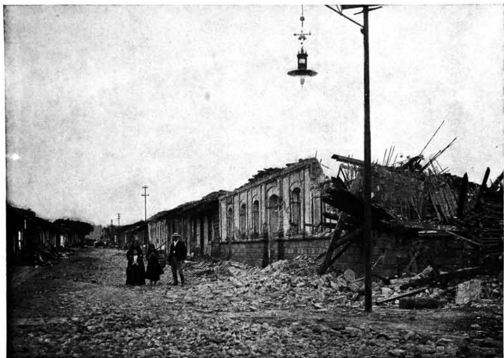
ONE OF THE PRINCIPAL STREETS IN CARTAGO AFTER THE EARTHQUAKE OF MAY 4, 1910
