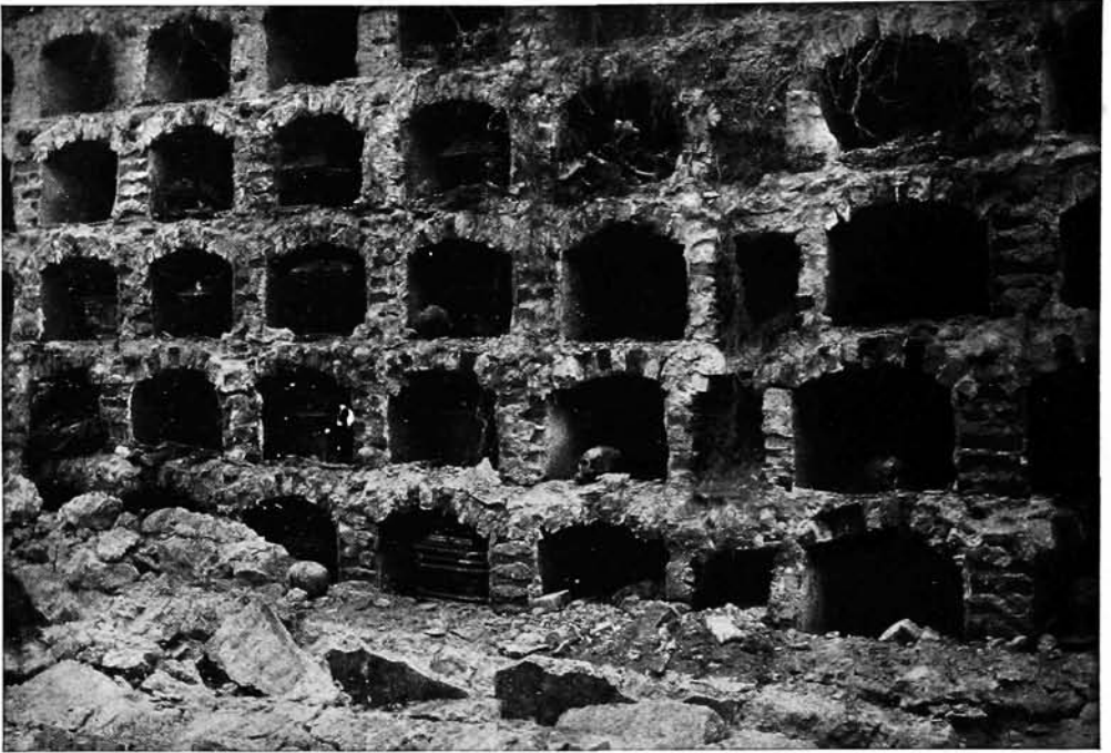
THE CEMETERY AT CARTAGO, SHOWING THE VAULTS BURST OPEN BY THE EARTHQUAKE
