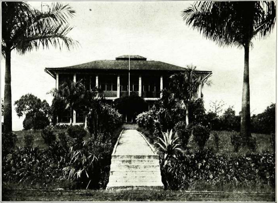
Chief engineer's house at Culebra, in which Colonel Goethals lived during the period of Canal construction. It has been removed and rebuilt at Balboa Heights, on the Pacific side, and is now the governor's residence.
