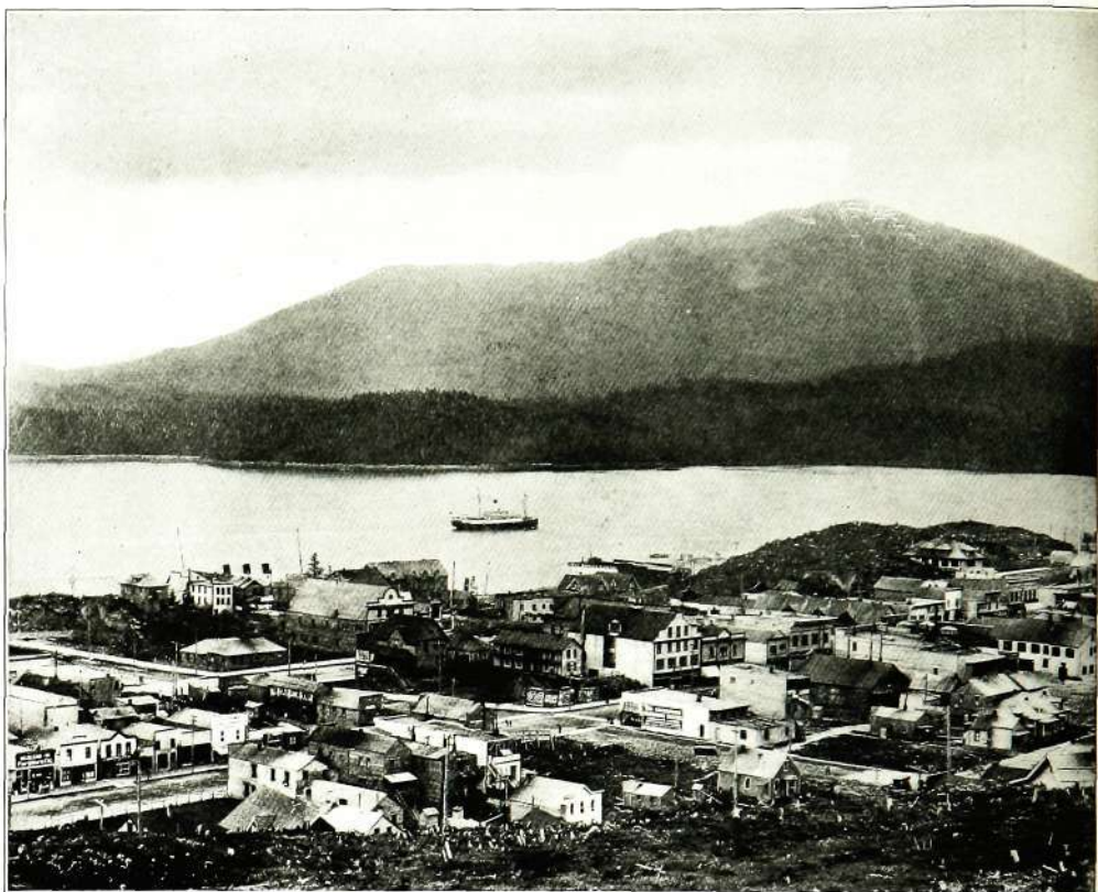
Prince Rupert, the western terminal
