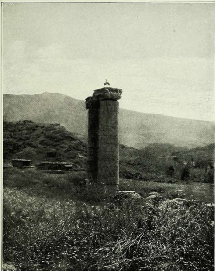
The columns before the excavations were begun, March, 1910.
