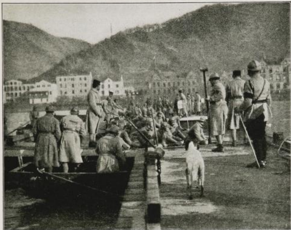
French soldiers pontooning the Rhine at St. Goar. Dropping the last pontoons into place.
