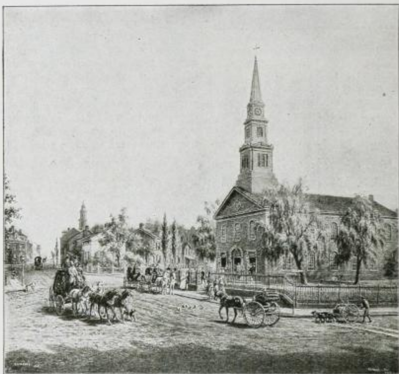
Old St. Marks-in-the-Bouwerie.
