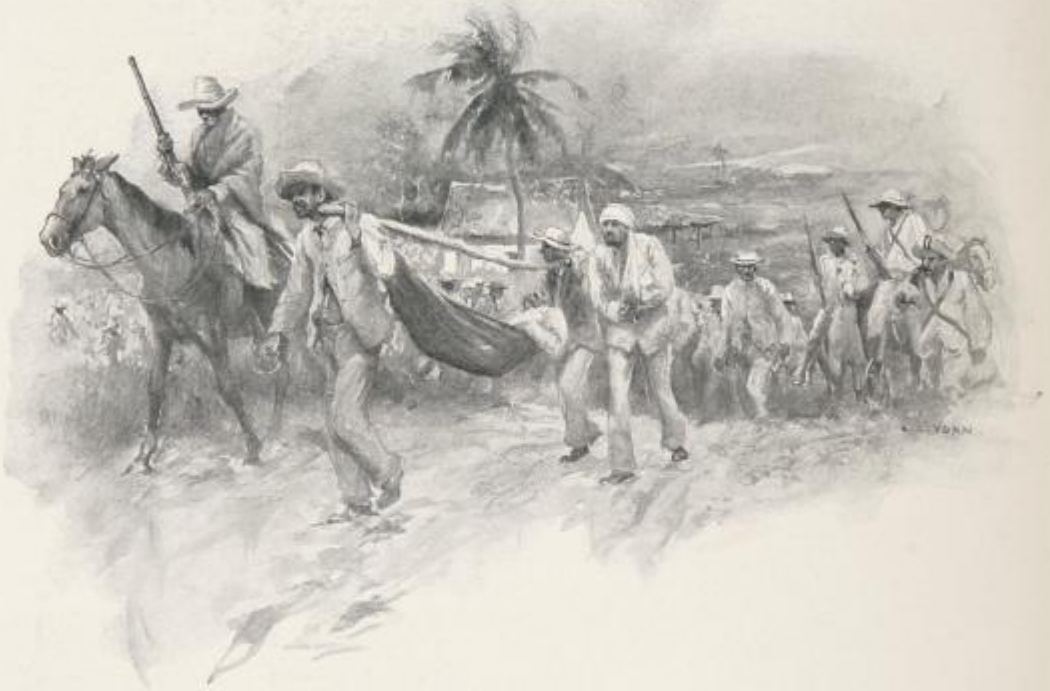
The march was painfully slow, the roads being in shocking condition.—Page 595.
