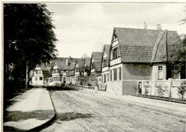
Some of the more pretentious houses in one of the Krupp colonies at Essen, Germany.
