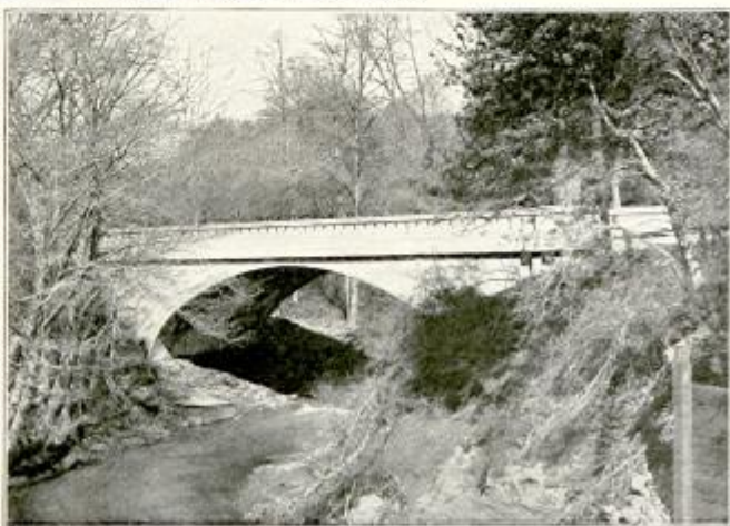
Reinforced concrete arch bridge. Constructed by the town of Ross, Marin County, California.
