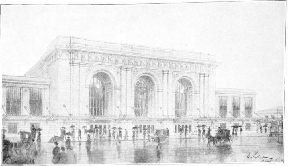
Approved design for the new station at New Haven, Connecticut. New York, New Haven and Hartford Railway.
