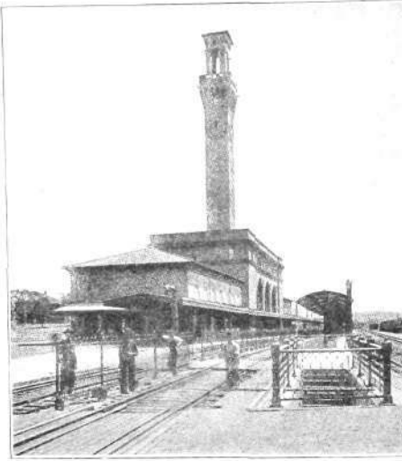
The new station at Waterbury, Connecticut.
