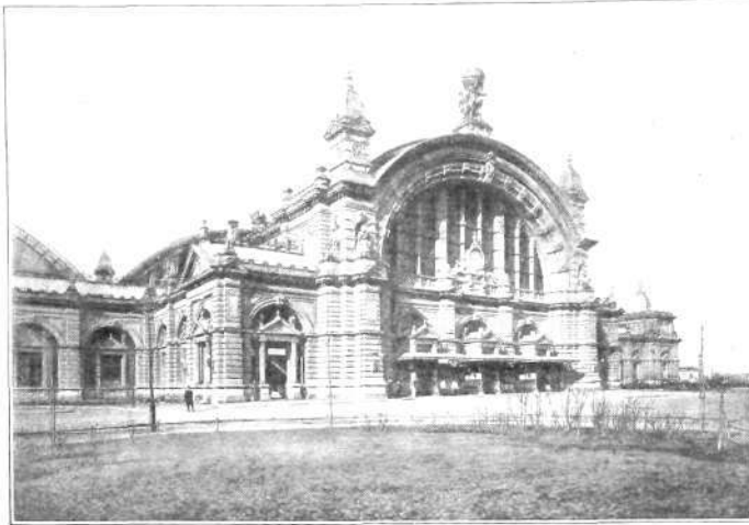
Frankfort Station, Germany.
