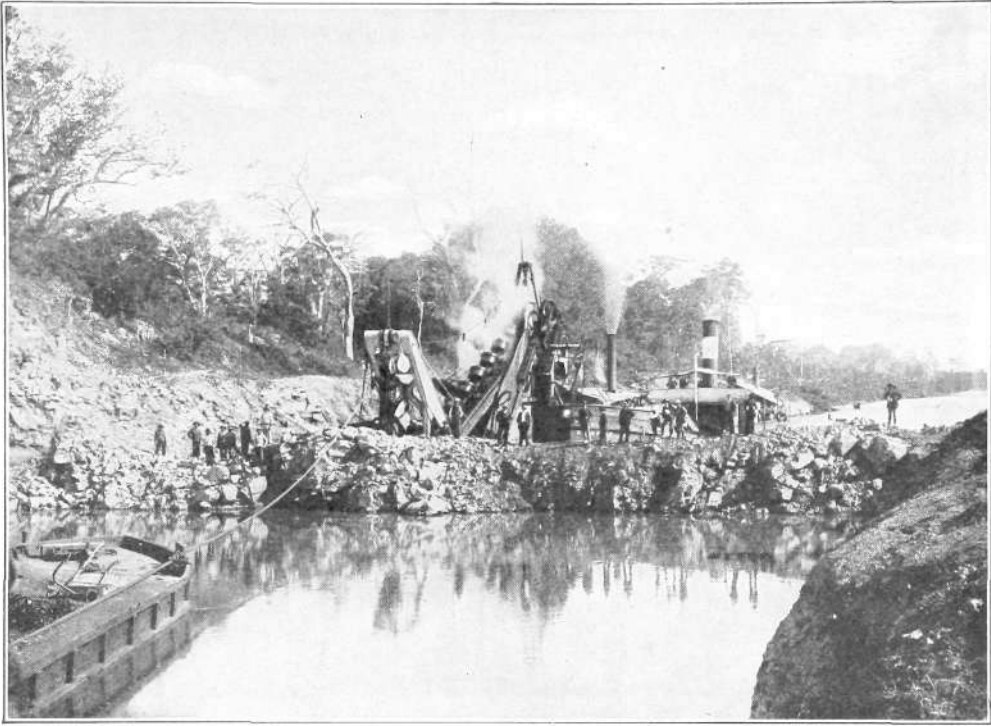
French dipper dredges at work in canal.
