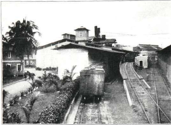
General view, cold-storage plant, Cristobal.
