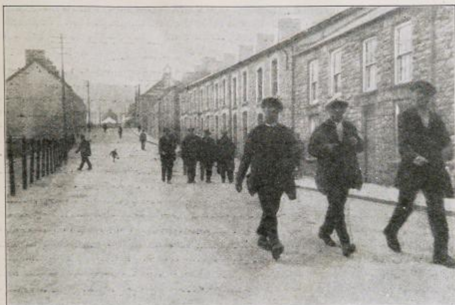
Miners returning from work in a coal town in the Rhondda district, South Wales.
