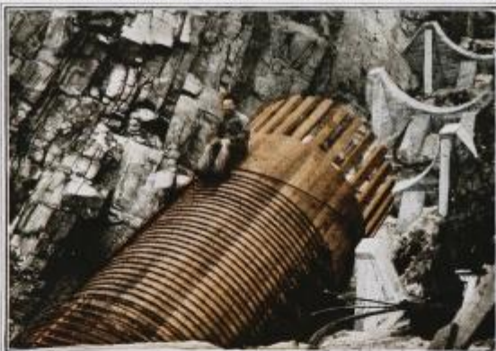
8 ft. inside diameter continuous redwood stave pipe built for the United States Reclamation Service, Sun River Project, near Gilman, Montana
