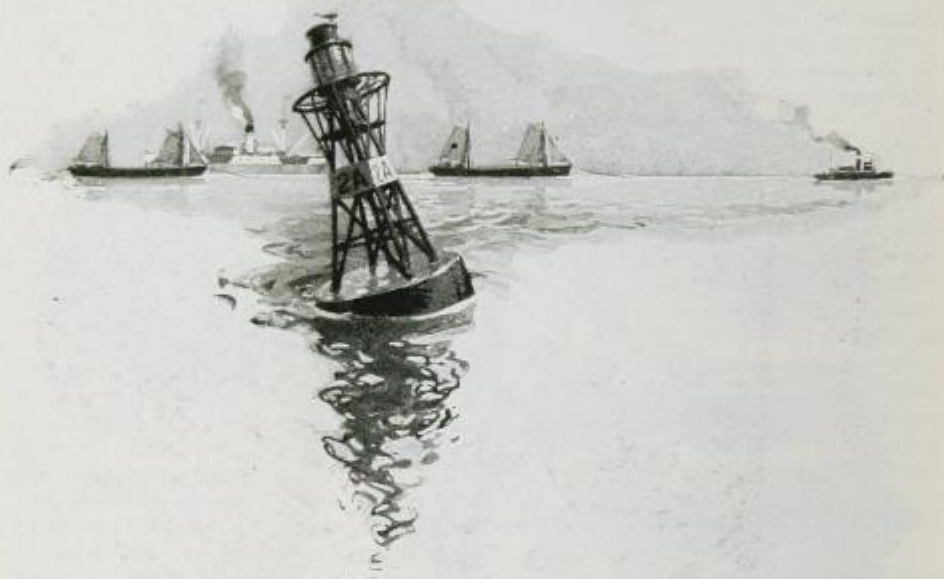
Sea-going barges outward bound passing a gas harbor buoy.
