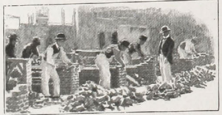
A class in bricklaying.
