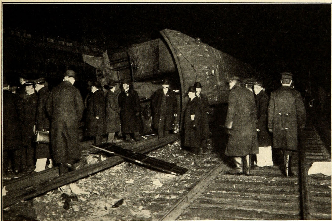
WRECK OF THE WHITE PLAINS AND BREWSTER EXPRESS IN 1907, ONE OF THE FIRST ELECTRIC TRAINS ON THE NEW YORK AND HARLEM DIVISION OF THE NEW YORK CENTRAL. 18 PERSONS WERE KILLED OUTRIGHT AND MORE THAN 70 INJURED, MANY OF THEM SERIOUSLY
