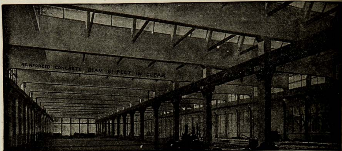
Interior view, before completion, of the immense Assembly Room (122 x 401 feet) of the Geo. N. Pierce Manufacturing Plant at Buffalo. Plant has over 325,000 square feet of floor space. Built complete according to the Kahn System of Reinforced Concrete.
