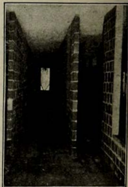
Interior view of above building, during construction, showing fire-proof partitions carrying fire-proof floor.
