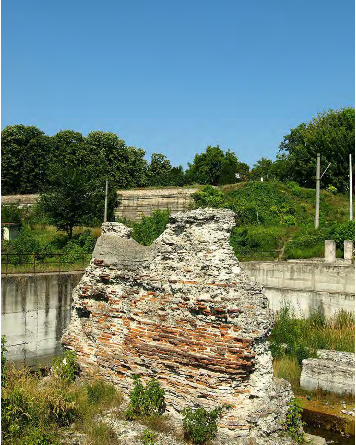
Figure 2.10 – Ruins of a pier of Trajan’s bridge on the Romanian shore of the Danube (at Drobeta-Turnu Severin, ancient Drobeta ). It is now surrounded by a concrete enclosure that was built to protect it from the rise in water level created by the construction of the Iron Gates 1 dam.
