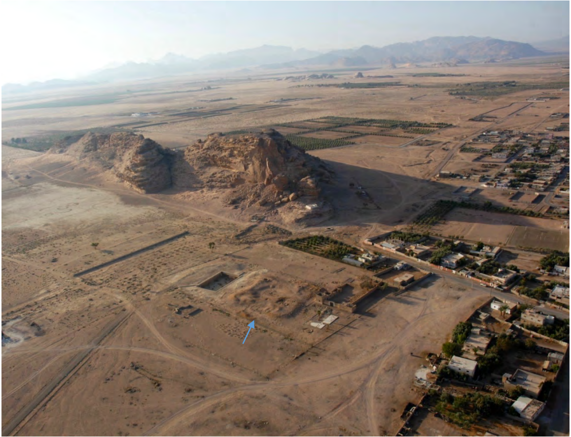
Figure 3.45 – Fort at Quweira, marked by a blue arrow in the foreground (Roman fort built over an earlier Nabataean structure).
