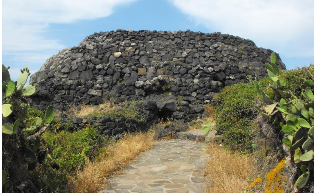
Figure 15: The Seso Grande in Pantelleria, located close to the Bronze Age village of Mursia, is a turreted-type structure with several entrances going around the structure. Several other sesi can be found immediately in this northern part of Pantelleria.
