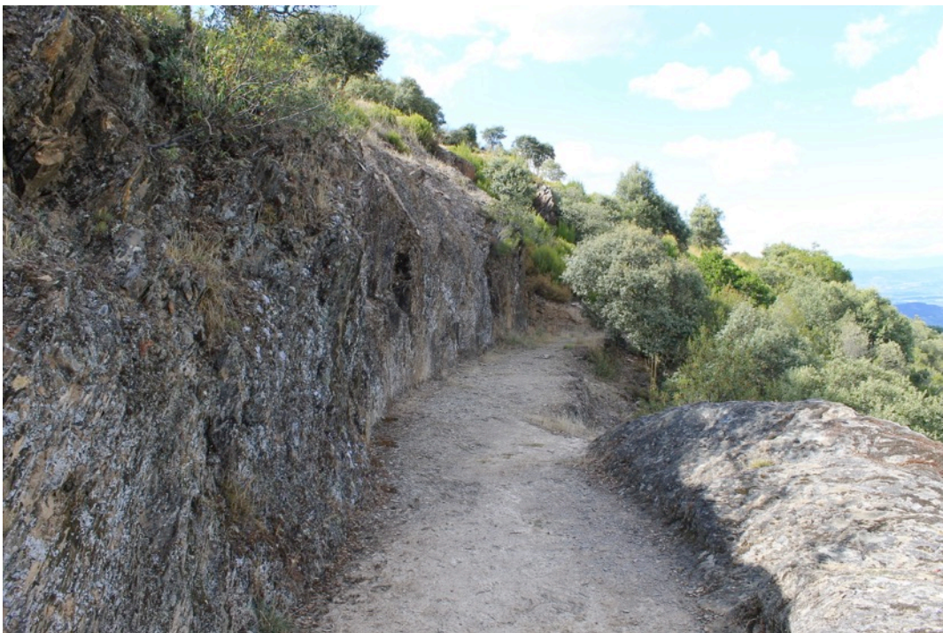
Figure 4.28 Corrugi or channels for directing water towards the tunnels excavated in the mountains (author photo).
