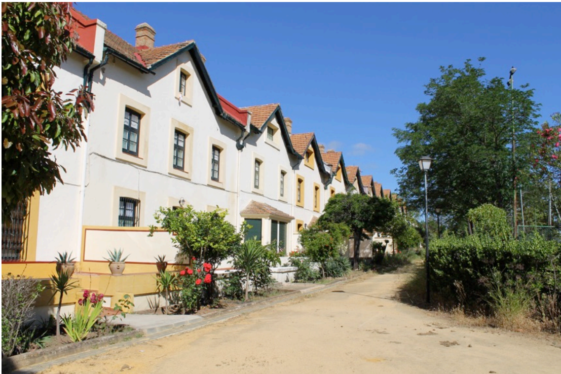
Figure 6.18 Victorian-style houses in the British neighborhood of Bellavista at Minas de Riotinto (author photo).
