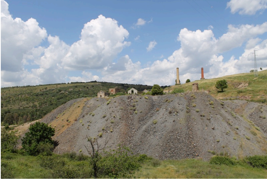
Figure 5.6 Contemporary mining installations at the well-known Roman mine of El Centenillo in Linares (Jaén, Spain) (author photo).
