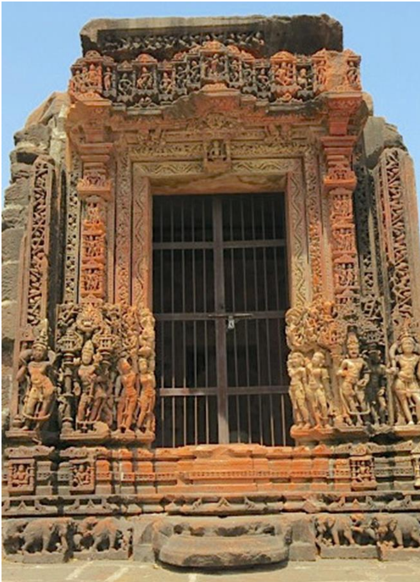
Figure 129. Close view of ancillary shrine (right side in Figure 64) with Lakulīśa in the central niche
