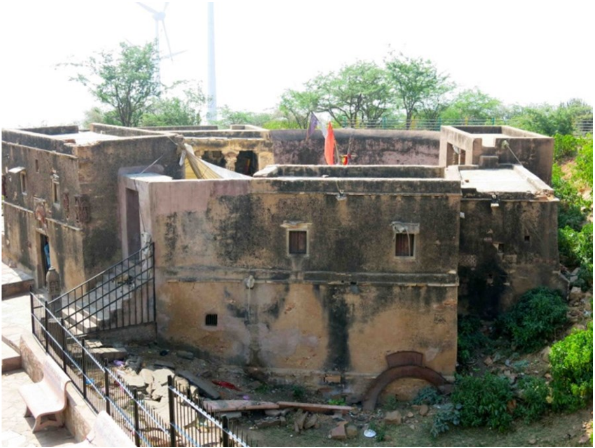
Figure 161. Renovated ma ha , now an active Bhairava shrine, Mt Harṣa Temple Complex
