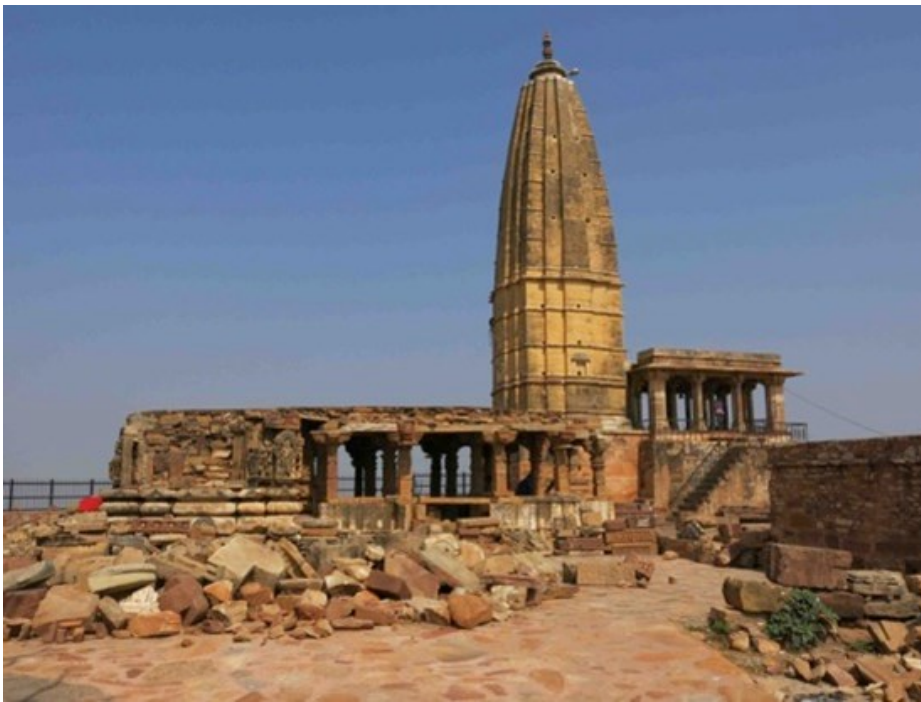
Figure 148. Remains of 10 th century temple on Harṣagiri (foreground)
