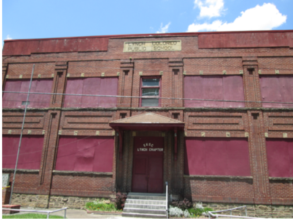
Figure 28. Lynch Colored Public School Building | 2014
