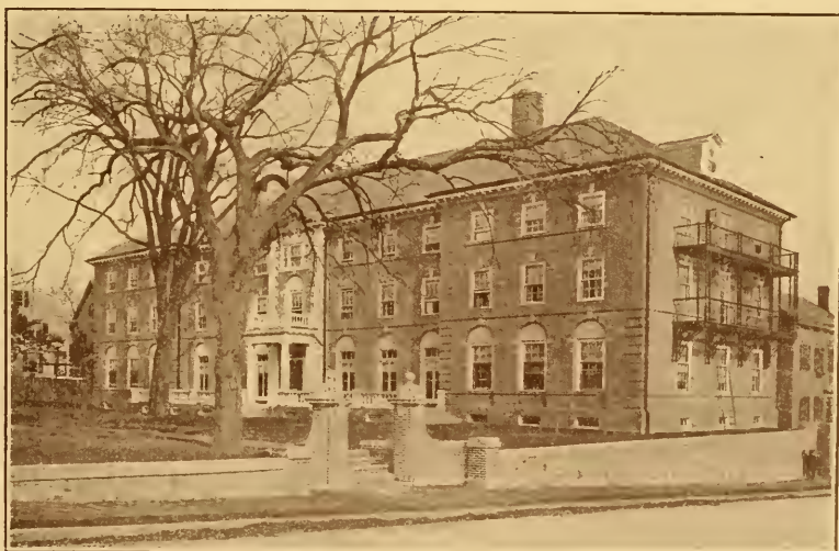
NEW HALL OF RESIDENCE, WOMEN'S COLLEGE
