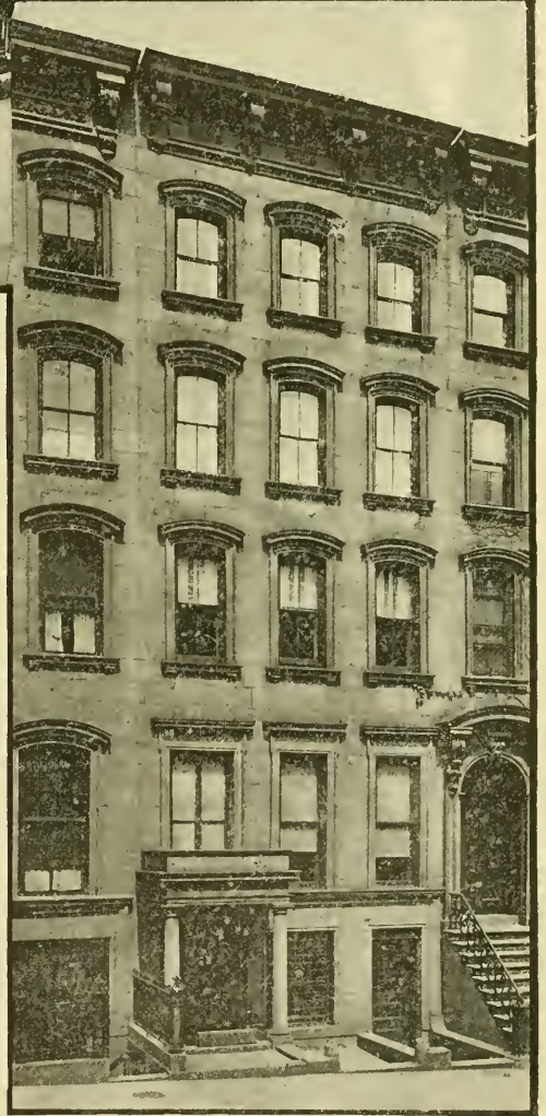
THE NEW BROWN CLUB 119 East 39th street
