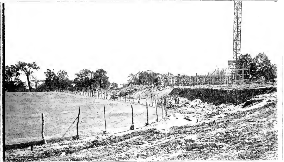
This picture, taken on September 24, shows the University gridiron at the left and the steadily rising stadium structure on the right
