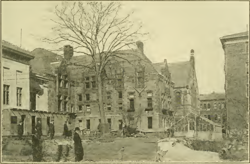
SITE OF ONE OF THE NEW DORMITORIES
