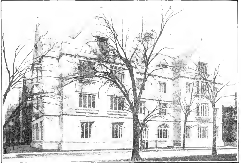
Classics Building University of Chicago. Built of gray Indiana Limestone
