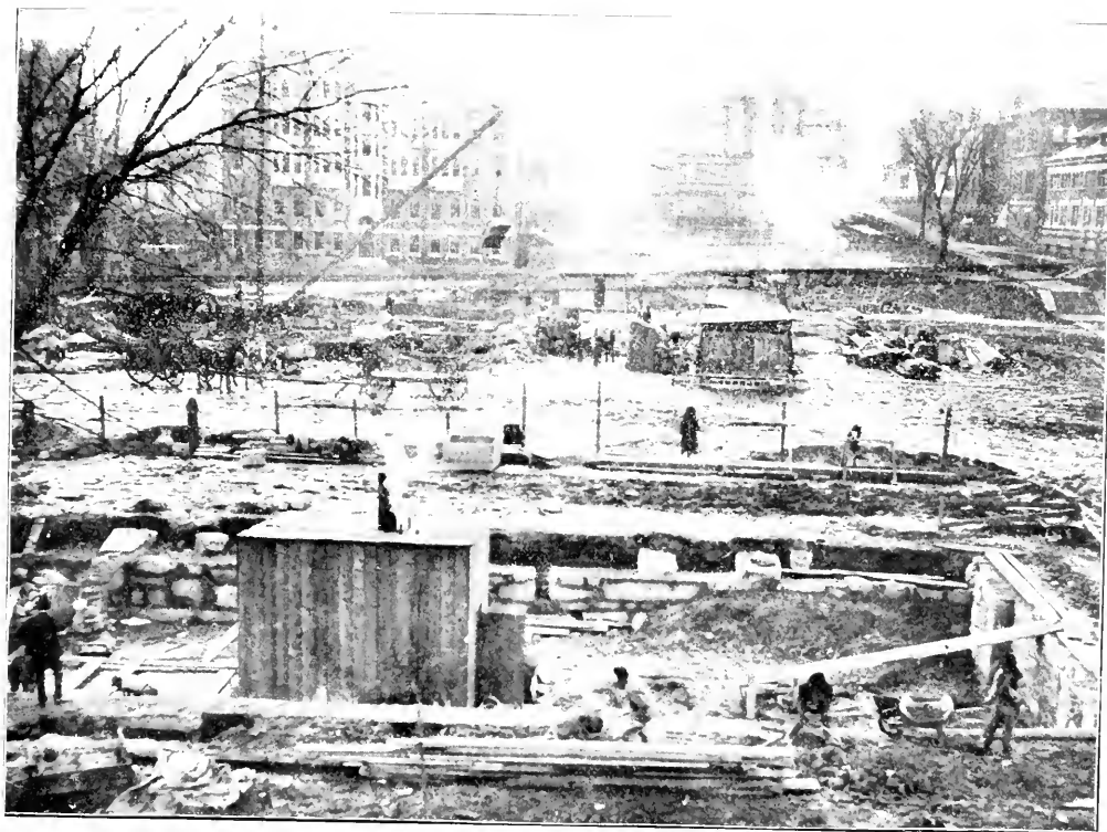
LOOKING WEST FROM BRUNOXIA HALL NEW DORMITORY IN FOREGROUND, ENGINEERING BUILDING BEYOND
