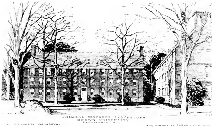
THE CHEMICAL RESEARCH LABORATORY: As envisioned by the architect. Its cornerstone was laid early this month.
