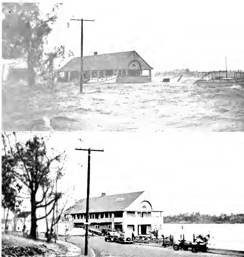
THE WATERS ROSE: At the height of the hurricane Roger T. Clapp '19 took the upper snapshot of the University Boat House on the Seekonk River. By comparing that furs with the other picture taken from the same spot after the river was normal again, one notes that the waters reached the second-story balcony, flooded the entire first floor where the fleet of dinghies is stored, and carried some of the river's motor boats up across the roadway. The flood picture, which shows the full violence of the storm, is the more remarkable in that it was 6:45 at night and vision was obscured by the flying salt sprays, some of which was carried inland as far as Woonsocket and beyond. The clubhouse and boats were in shape again in time for the annual alumni-undergraduate regatta on Alumni Day.
