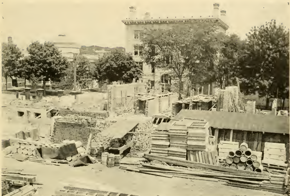
THE NEW DORMITORY ON THAYER STREET
