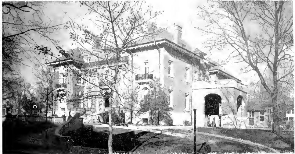
▲ SOUTH HALL, at right, first and still central building on the new Bryant campus, is one of 22 which would be offered to Brown. Many alumni will remember it as Hope Hospital.
