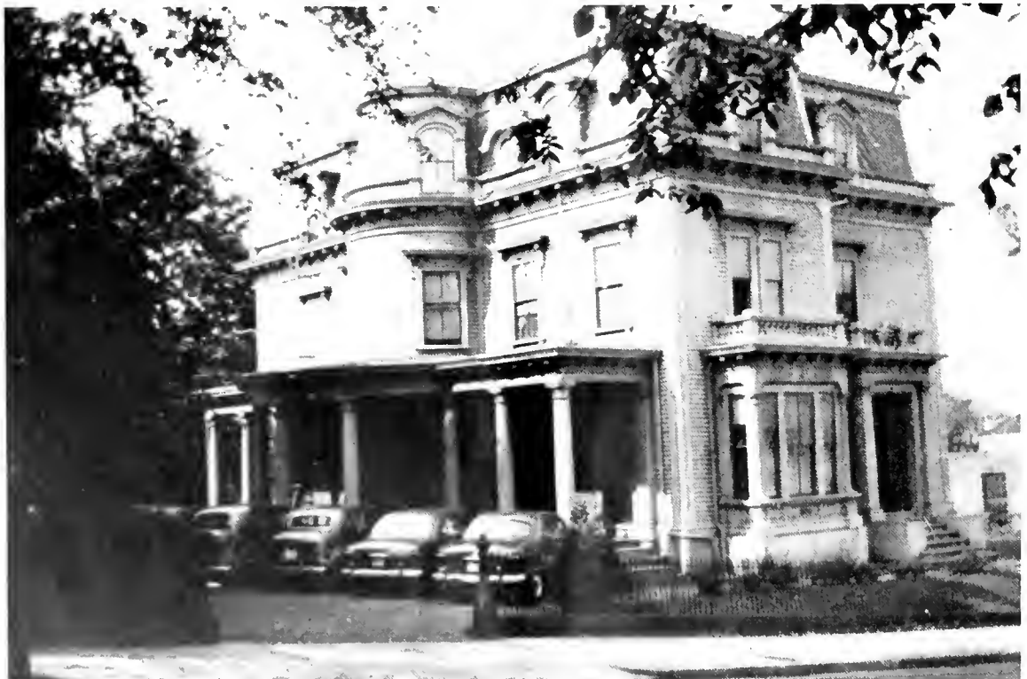
IN THE WRECKER'S HANDS: The former Phi Kappa Psi House at Brown was being razed in January, the site to be used for parking by the University Club.
